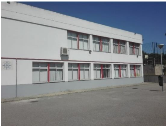
Figure 25 – Administrative pavilion , east façade. Source: Google Earth Pro; year: 2018
